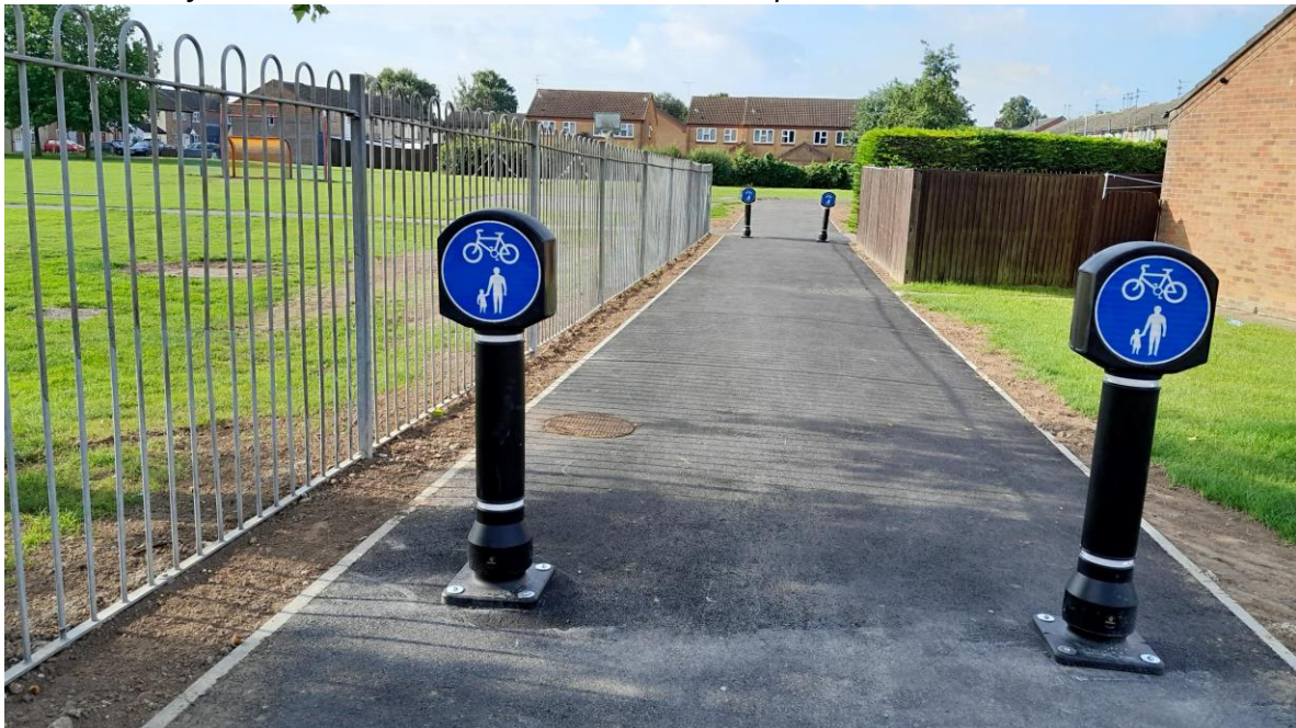
Installation of bollards between road access and Skatepark
