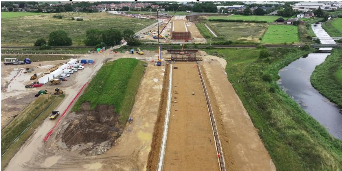
SWRR – Aerial Progress Photo in August 2023 looking east
