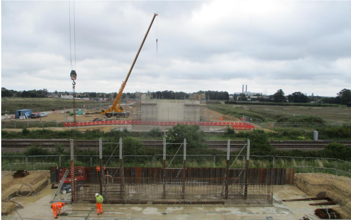
SWRR – Steel fixing to west pier
