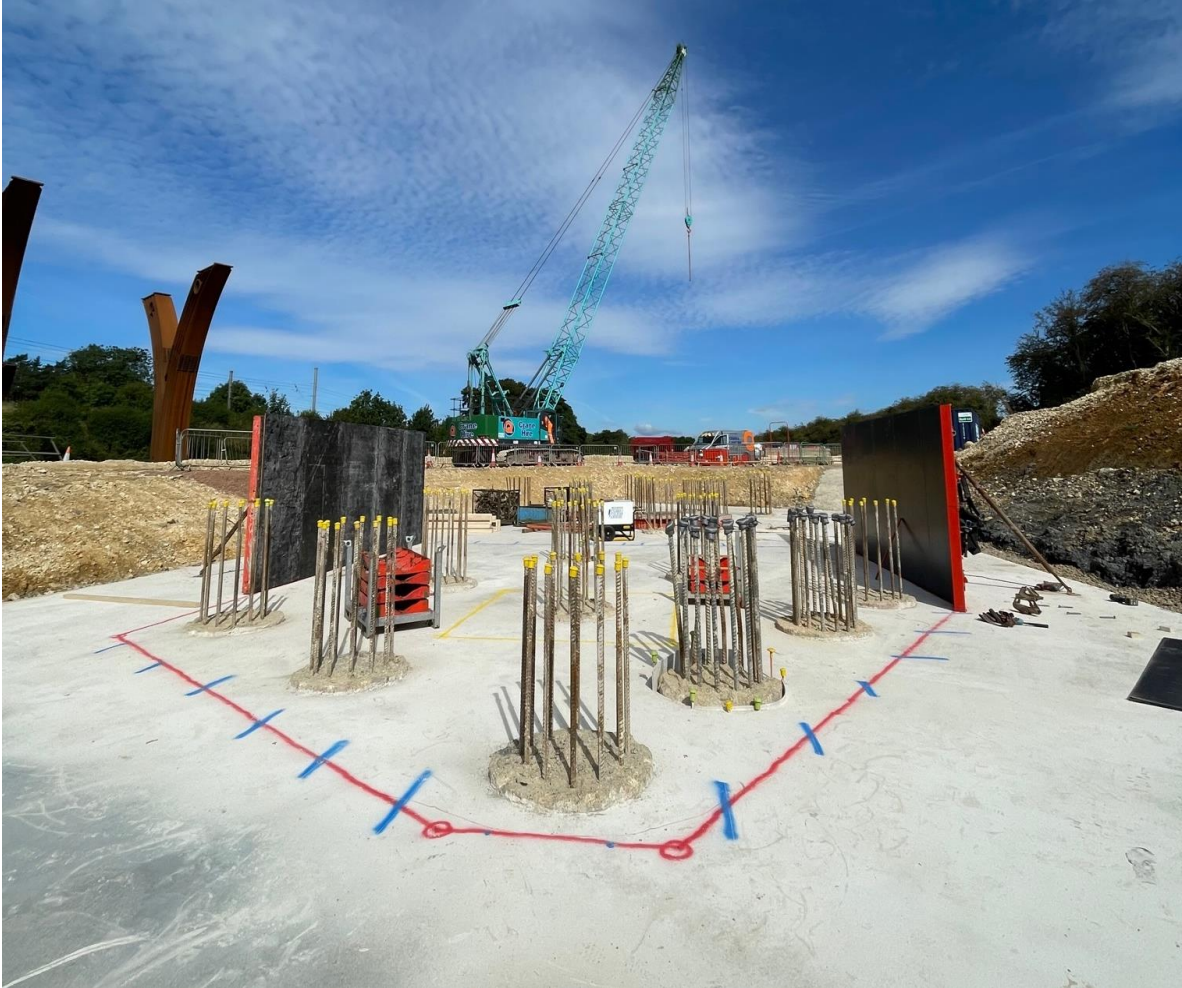
GSRR – Pier 5 Cropped Piles
