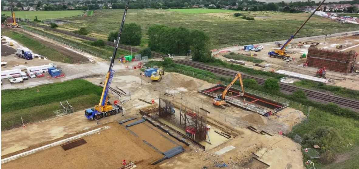
SWRR – Aerial Progress Photo in August 2023 looking north east
