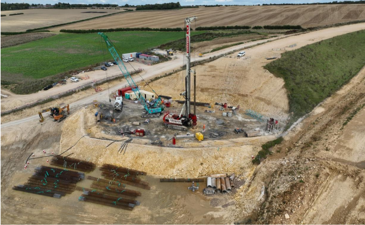
GSRR – Piling Operations for Eastern Abutment
