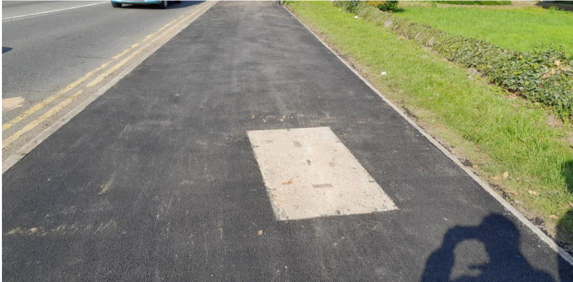
Completed section on north side of A151
